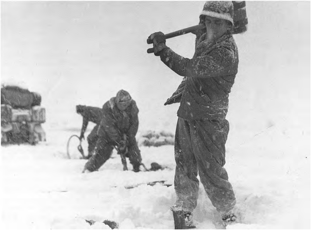
BUILDING DEFENSIVE WORKS IN THE SNOW. 111th Engineer Battalion, 36th Division, in Weibruch area.
