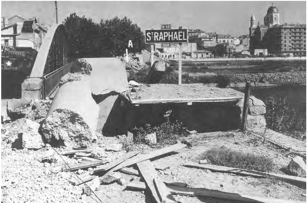
PILLBOX GUARDS BRIDGE TO ST. RAPHAEL. Supporting installations are behind it.
